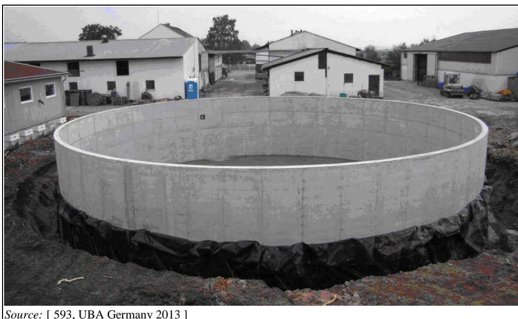
Figure 4.79: Underground slurry tank with liquid-tight geomembrane
