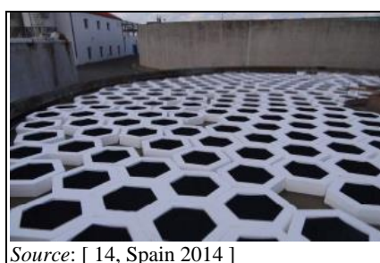
Figure 4.78: Geometrical plastic tiles in a slurry tank
